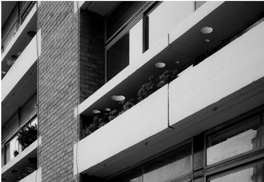
Photo of Cullum Welch House pre-cast concrete planters at floor and cill level, highlighting the holes for flower pots.
