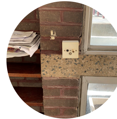
Exposed aggregate concrete
