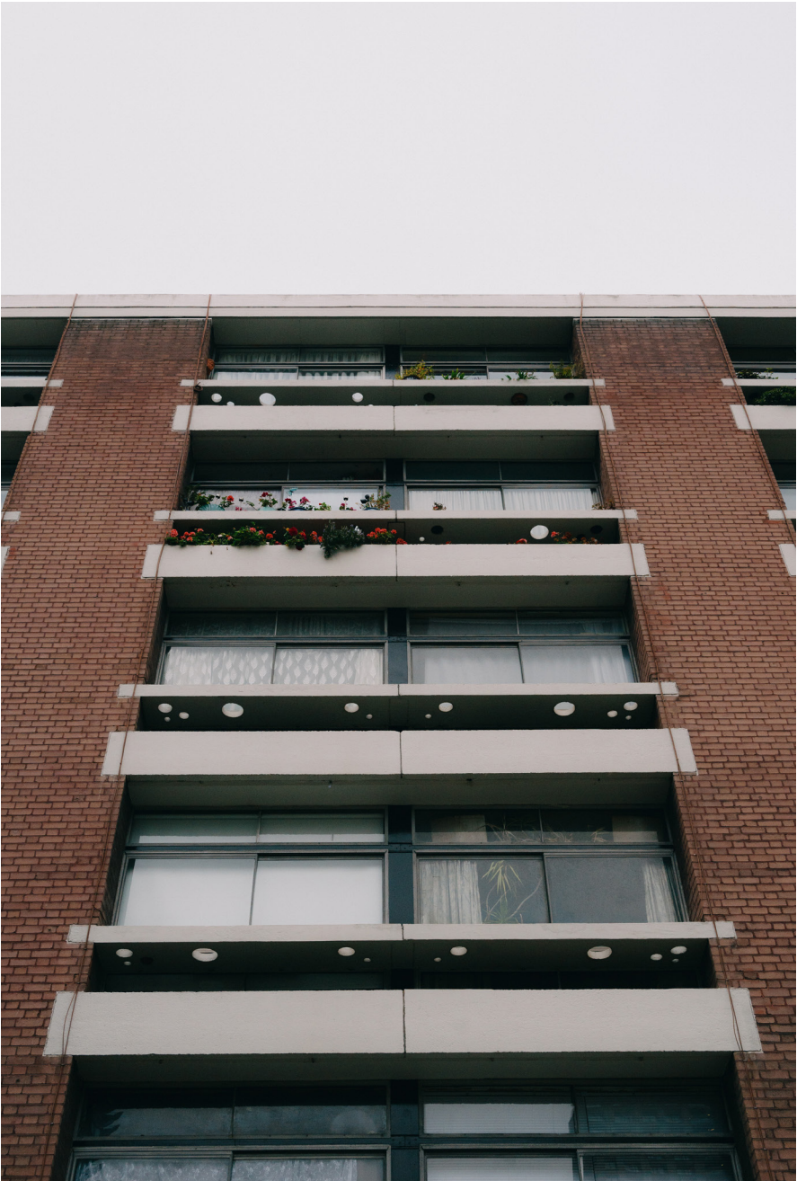
Photograph of Cullum Welch House, showing the fully glazed south elevation and pre-cast concrete planters at floor and sill level, highlighting the holes for flower pots.
