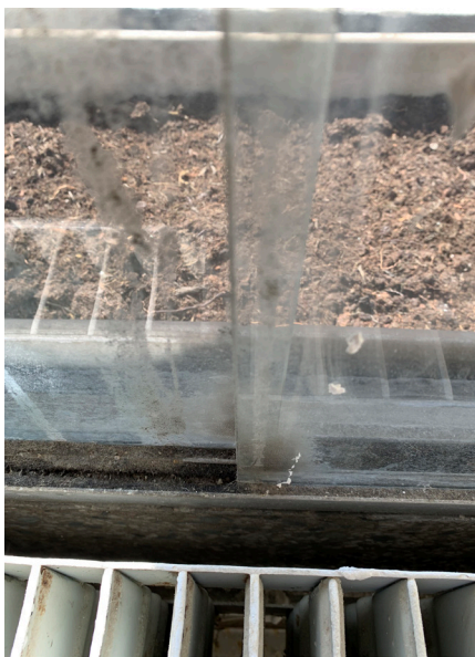
The original sliding aluminium bar appears to be missing on some of the unframed sliding windows, leaving a gap for warm to escape out of.
