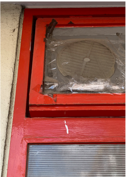
Ventilation panels have been retrofitted into some windows and some have subsequently been covered to stop any draughts.
