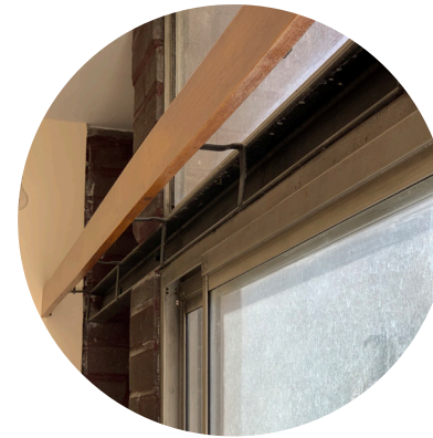
Timber curtain rail and steel C-section
