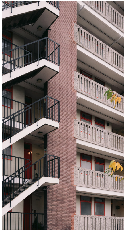
Photo of Cullum Welch House northern facade, highlighting the tomato red painted timber windows and the open access concrete balconies.
