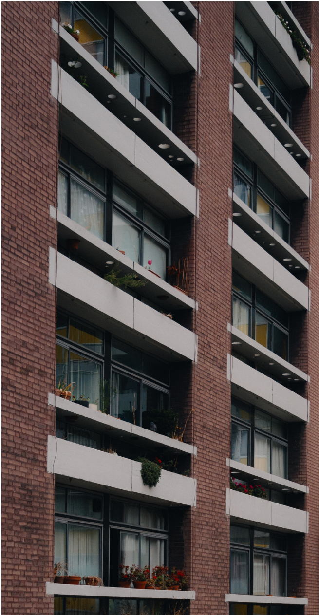
Photograph of Cullum Welch House, showing the fully glazed south elevation, pre-cast concrete planters at floor and sill level and brick piers.
