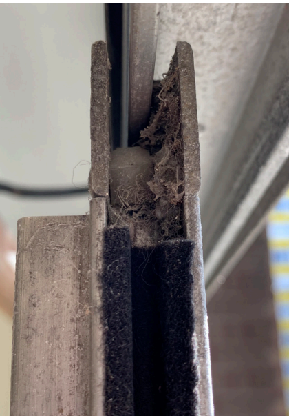
The original aluminium frames and runners are weathered and stiff, showing signs of oxidation.
