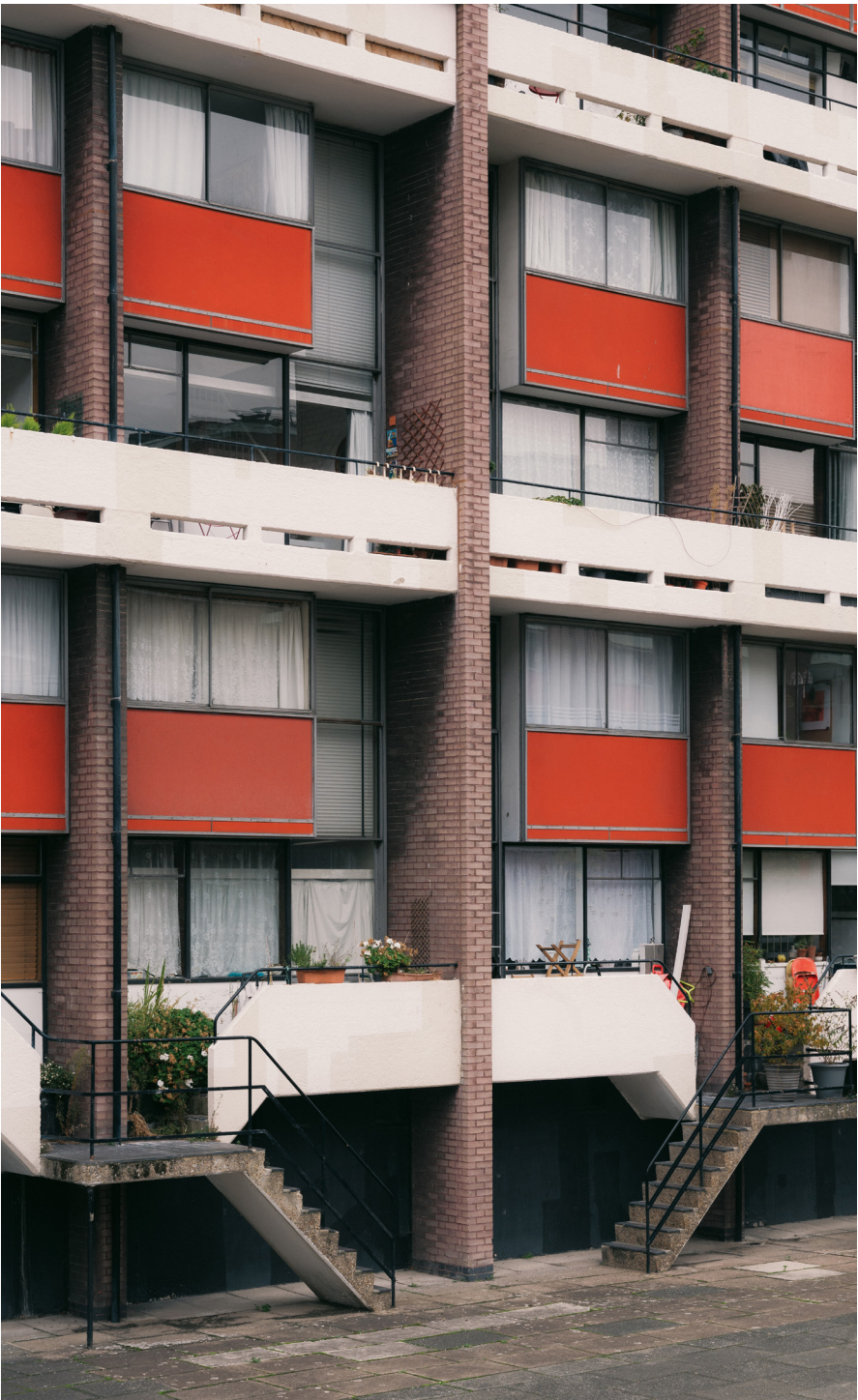
Photograph of Basterfield House, highlighting balconies and private stairs, red Muroglass spandrel panels and glazing
