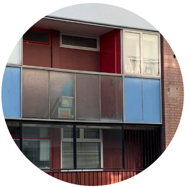
Right: a number of timber windows look to have been replaced with uPVC windows, confirming issues with condition or thermal comfort, or both.
