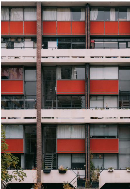
Photo of a section of the south facing side of a typical maisonette block. Dependant on the building, these face the road or a shared courtyard and the Muroglass cladding is red or blue.
