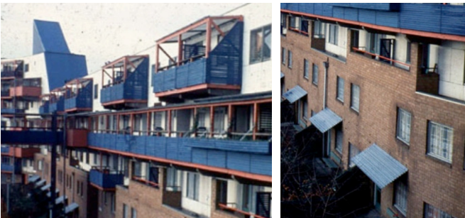
Byker Wall (Newcastle Upon Tyne): Photo of existing window/façade treatment (left) and new, replacement windows/façade works, including steel balcony structures (right).
