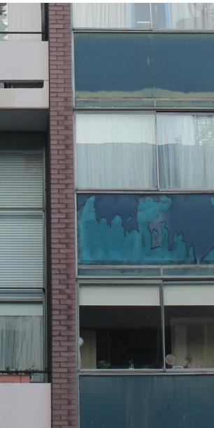
Damage/deterioration of the Muroglass spandrel panels. Many are faded or have been replaced with a poor colour match
