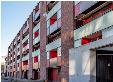
Photo of Basterfield House north elevation, highlighting decked access and escape balconies
