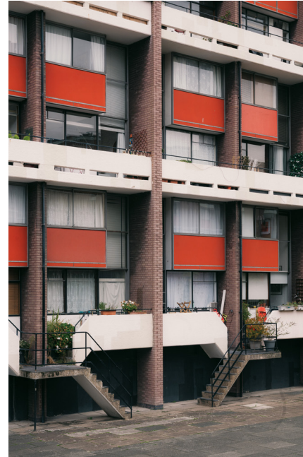
Photo of Basterfield House south elevation, highlighting one type of the concrete steps to courtyards
