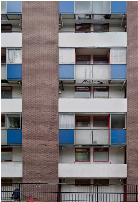
Photo of a section of the north facing side of a typical maisonette block. Dependant on the building, these face the road or a shared courtyard and the Muroglass cladding is red or blue.
