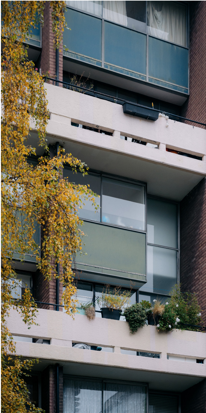
Photograph of Hatfield House south elevation, showing the projecting bedrooms with horizontal sliding windows, guillotine door/window system, balconies and brick piers.
