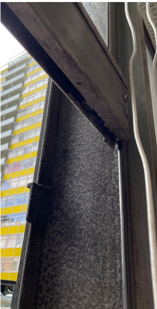
Oxidisation of the aluminium frames internally and externally (door system)
