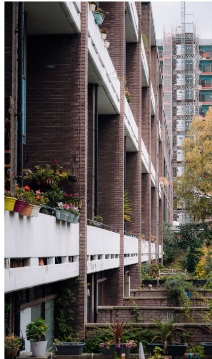
Photo of Hatfield House south elevation, highlighting brick cross walls projecting at either end of the balconies and small gardens
