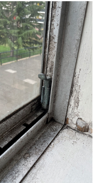
Oxidisation of the aluminium frames internally and externally (sliding). Peeling paintwork to timber reveal
