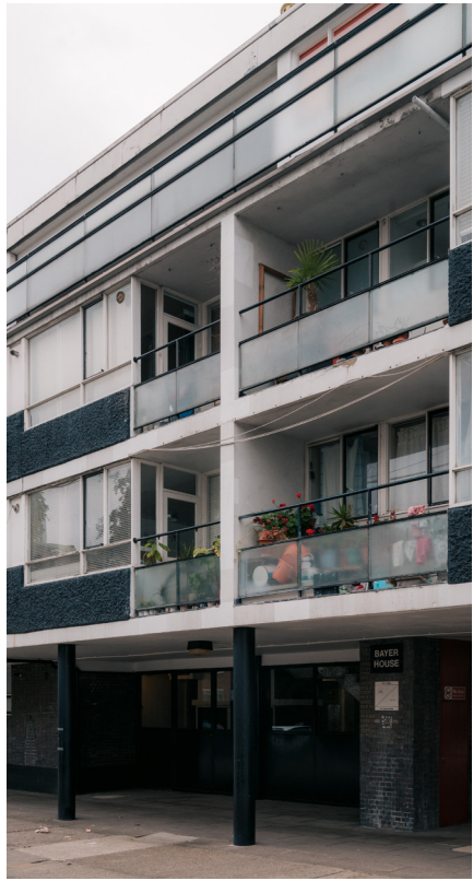
Photo of Stanley Cohen House east elevation, facing Golden Lane. Inset balconies to 1st, 2nd and 3rd floor, with the colonnade running at ground floor next to the road.
