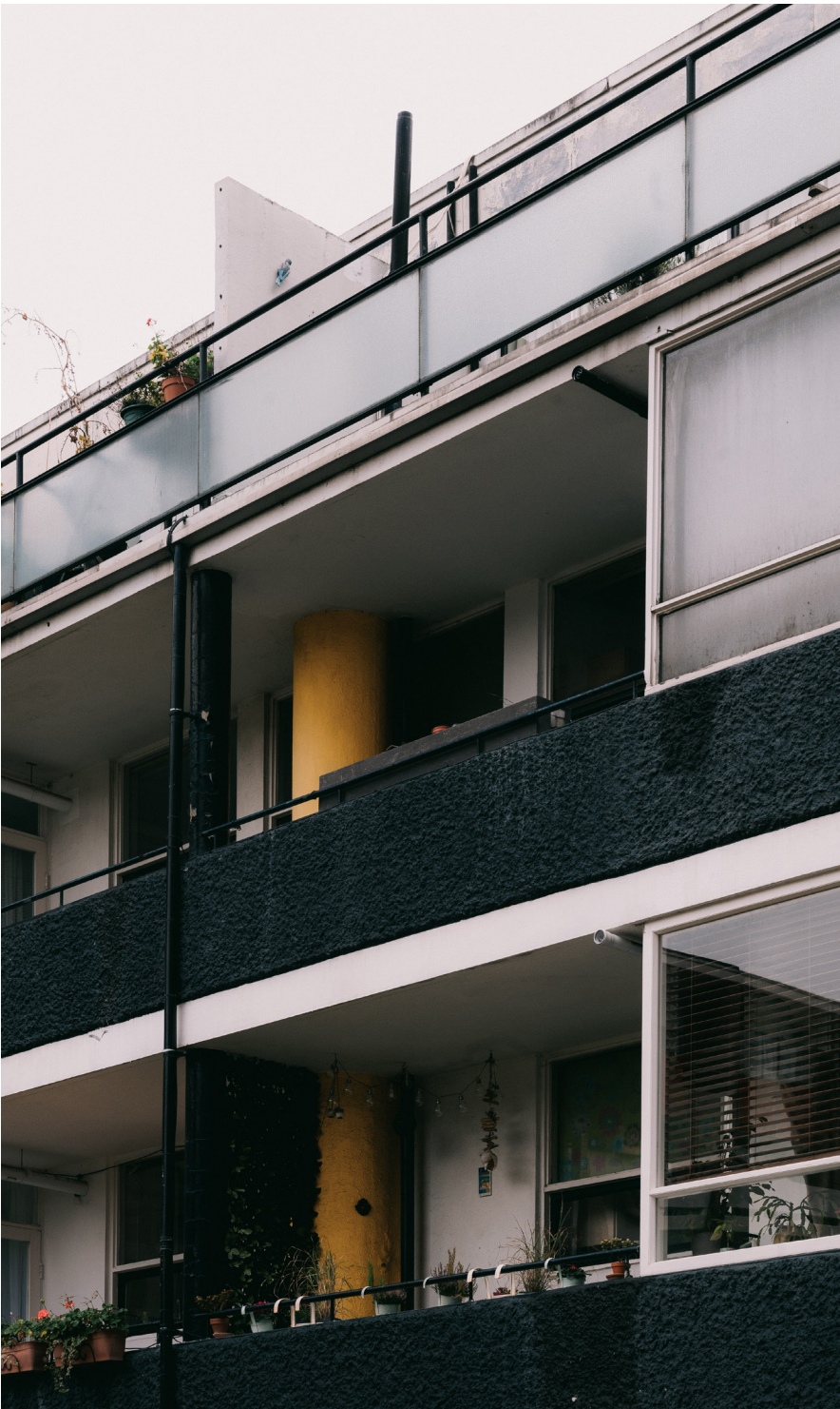
Photograph of Stanley Cohen House West elevation, highlighting balconies, yellow bin chutes and glazing.
