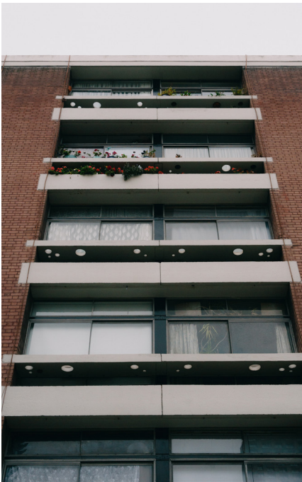
Photo of the outward facing Cullum Welch House elevation, capturing details such as the pre-cast concrete planter holders.
