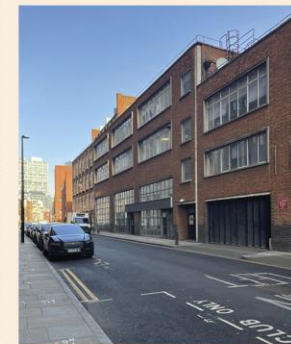
Existing facade to Goulston Street
