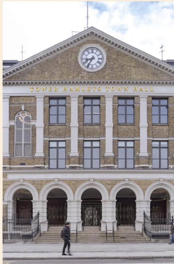
Tower Hamlets Town Hall - AHMM
