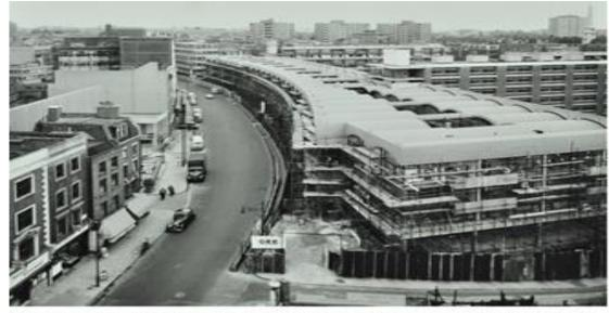
Certain parts of Crescent House were made off site whilst others were jointed on site. The frames and the concrete structure meet with no obvious details to accommodate tolerances, suggesting that a high level of custom sized joinery exists in the façade of Crescent House.
