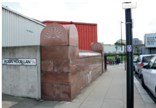
NORTHERN TUNNEL PORTAL PARAPET
