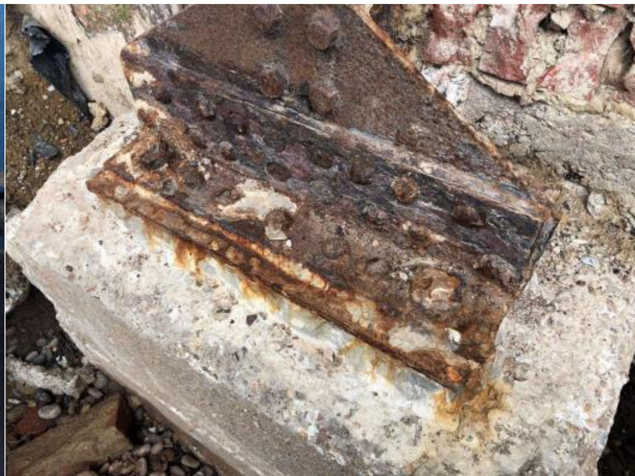
View of baseplate showing corrosion and missing rivet heads
