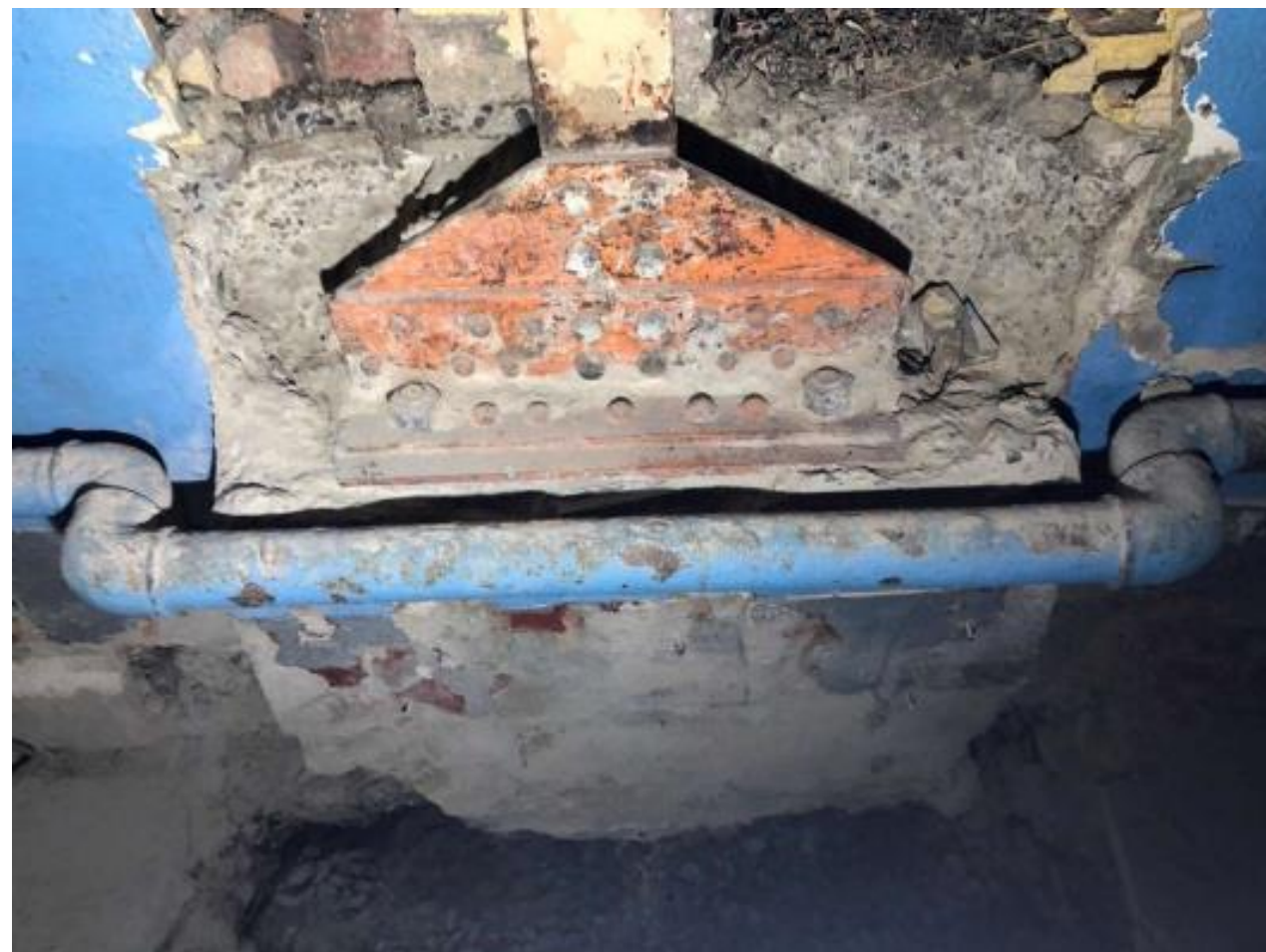
View of column baseplate into plinth (internal)
