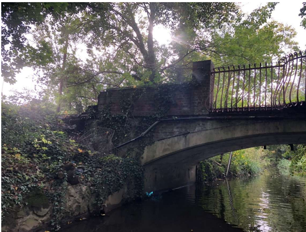
Figure 8 View from the river showing staining, water seepage and vegetation growth along arch, east of the bridge
