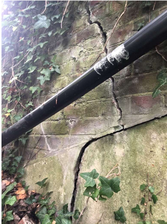
Figure 9 Cracking at arch springing at the south abutment on the east face
