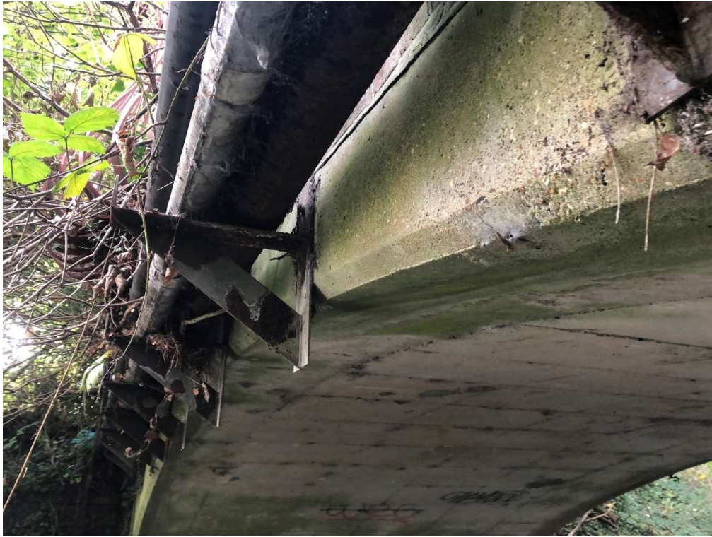
Figure 11 Corrosion at the steel brackets supporting ducts, west face of the bridge
