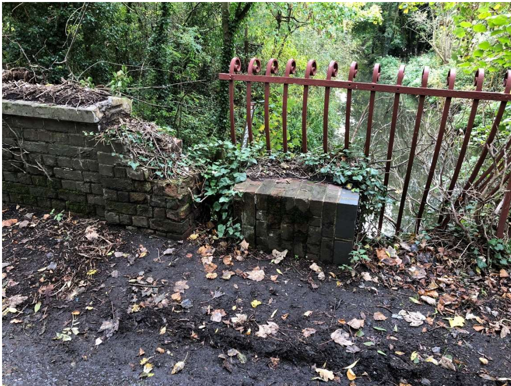
Figure 6 Longitudinal displacement of parapet on the western face, south of the bridge
