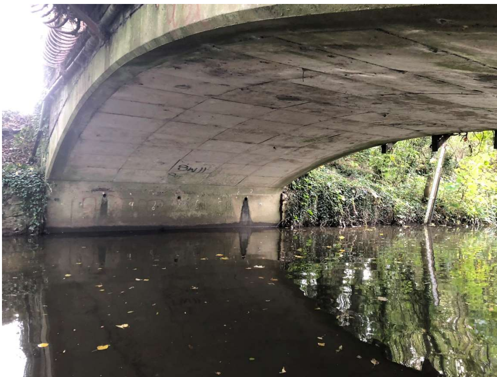
Figure 10 Soffit of arch on the east face showing minor spalling and staining
