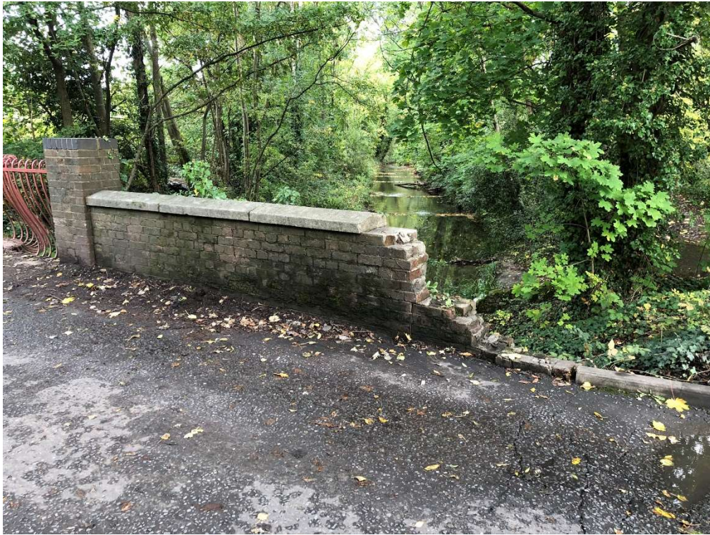
Figure 5 Loss of masonry at eastern face of parapet, south of the bridge
