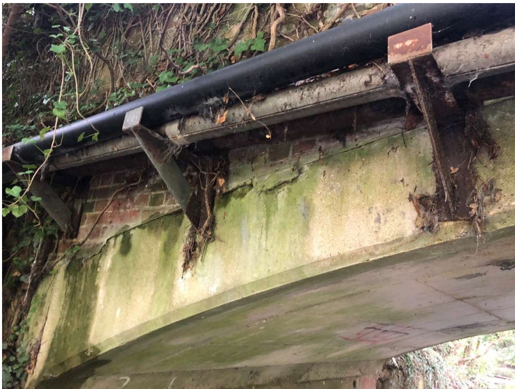
Figure 12 Water seepage at the arch-masonry interface, west face of the bridge
