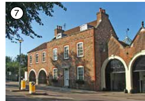
7 Devon House, Church Hill (Grade II)
