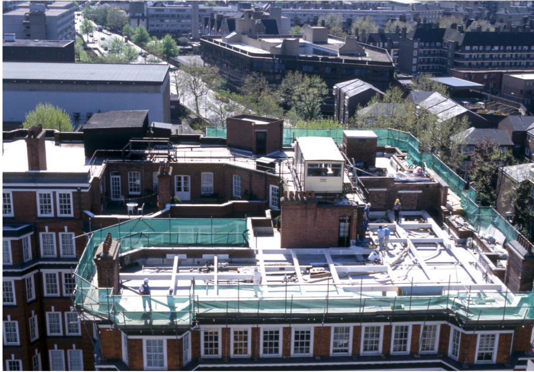
Parapet Scaffolding Only - St John's Wood Court
