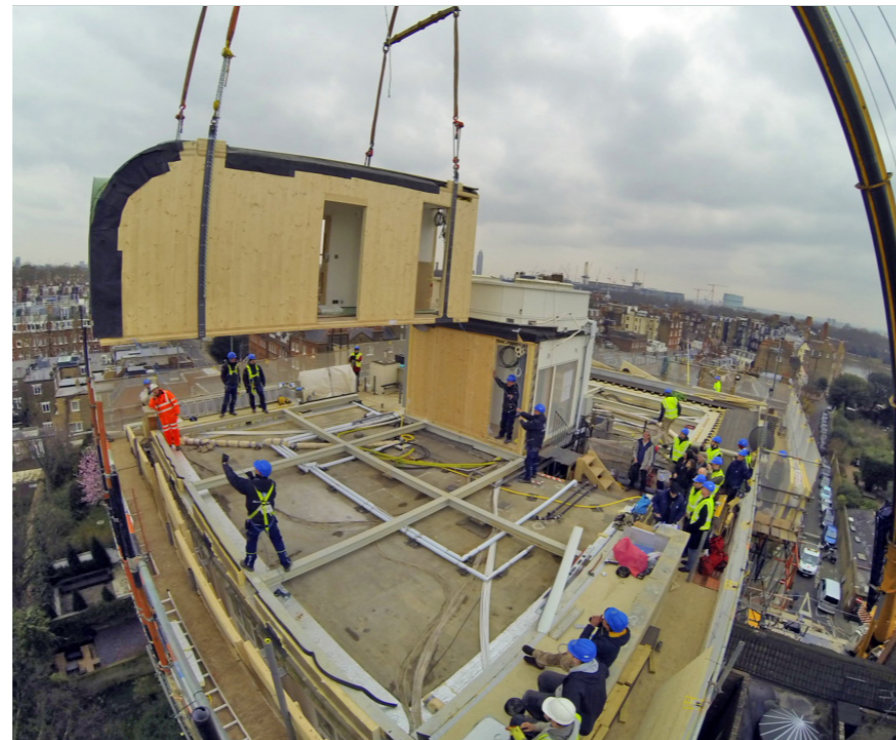
Module Delivery and Craning
