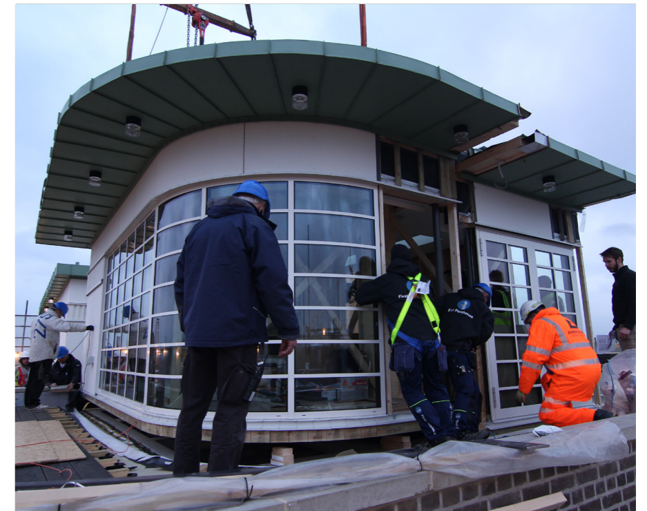
Precision Locating of Module
