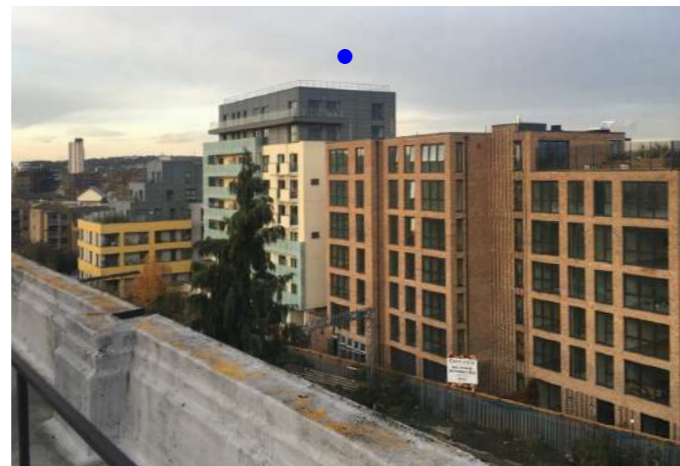
Centric Close from the Roof of Darwin Court, the Lock-house behind
