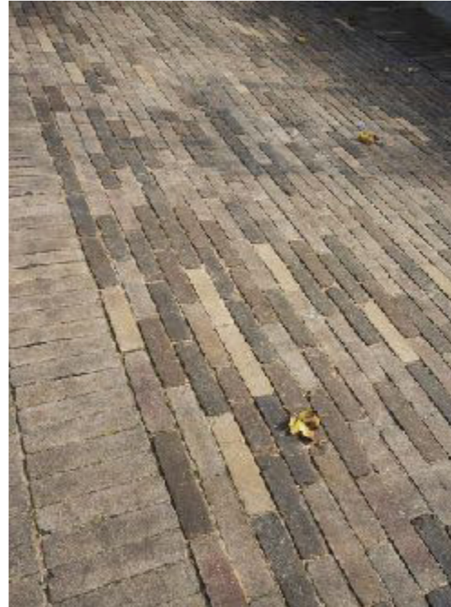
Flemish clay pavers to be used to form the new wide entrance paths to each of the five blocks.
