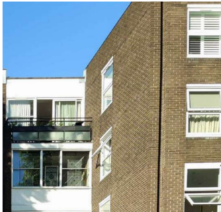
Windows in brick panels contrasting with light coloured panels with larger glazed areas.
