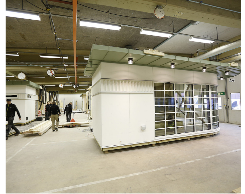
Modules Constructed in Factory Environment
