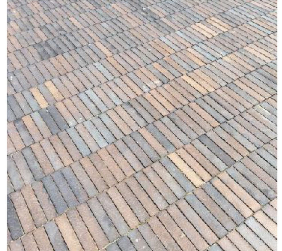
Flemish clay pavers to be used to form the new wide entrance paths to each of the five blocks.
