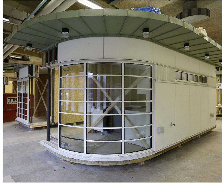
Modules Constructed in Factory Environment
