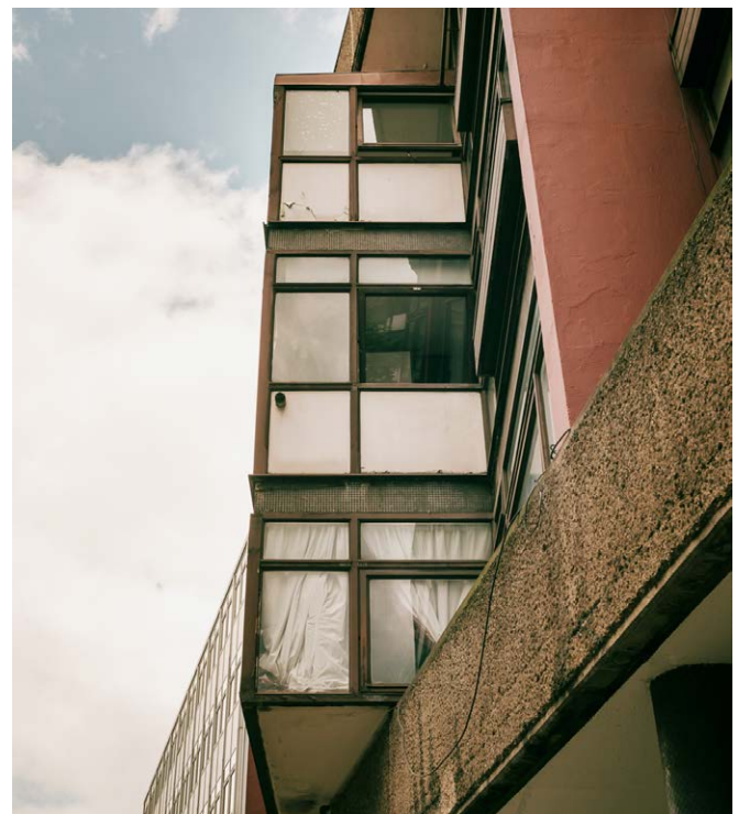
The west elevation projecting oriel windows, facing Goswell Road.
