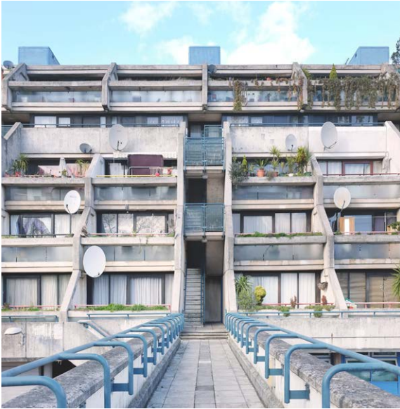
Alexandra Road Estate ahead of glazing replacement works.
