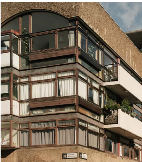
Crescent House South-West corner, showing the 2-bedroom flats and concrete balconies.
