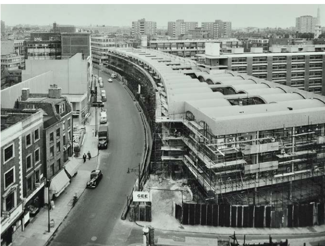
Certain parts of Crescent House were made off site whilst others were jointed on site. The frames and the concrete structure meet with no obvious details to accommodate tolerances, suggesting that a high level of custom sized joinery exists in the façade of Crescent House.
