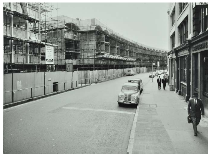
The photographs above show Crescent House under construction from Goswell Road.
