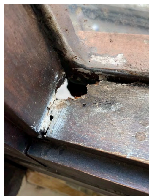
Deterioration of the hardwood frame/cill on the west façade where the glass pane has become exposed to the elements. Evidence of mould growth.
