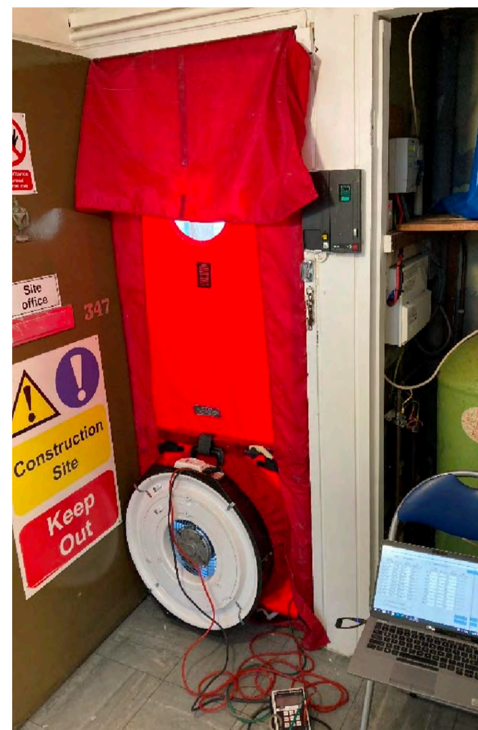
Above: blower door test equipment mounted in the front door
