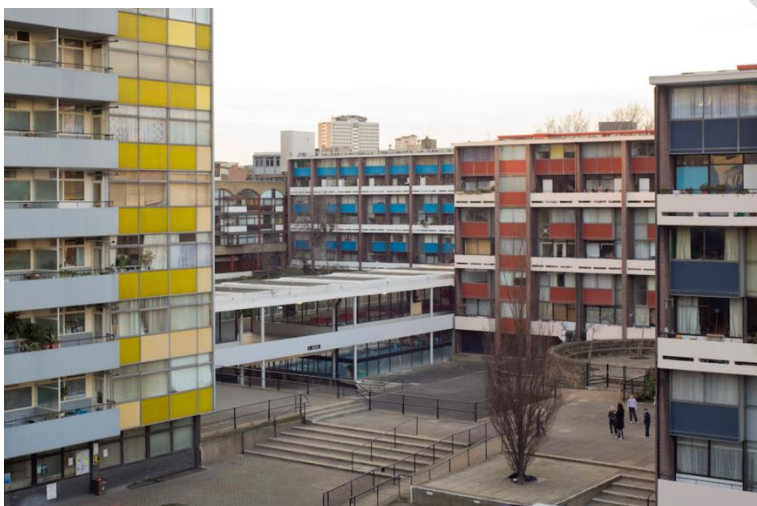
Figure 1: Golden Lane Estate
