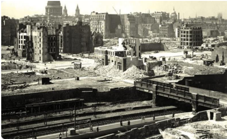
Figure 6: View south over Aldersgate to St Paul's
