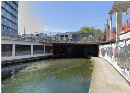
Current condition - deck over canal adjacent Camden Street bridge
