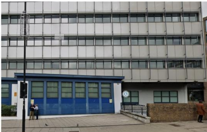
(D) Brick wall, railings and dated extension, Camden Road
