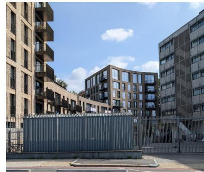
(F) View from Camden Street towards the canal, storage cabin blocking the view of the canal
