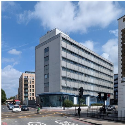
Existing Camden Road / Camden Street junction
