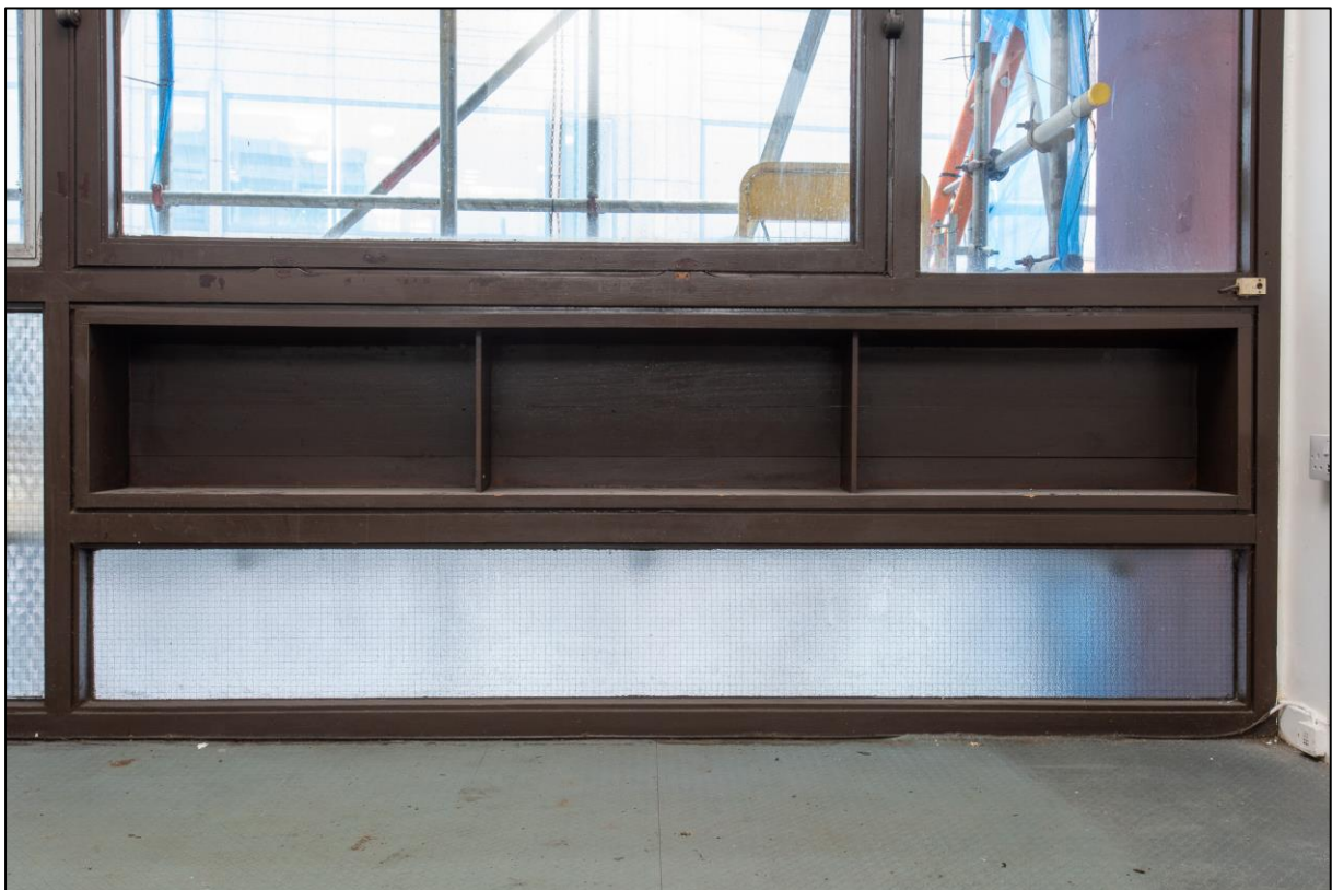
Figure 18. Bookshelf and fixed window with reinforced glass, looking west
