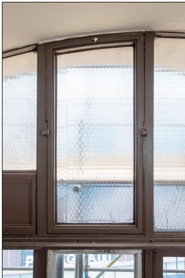
Figure 12. Central pivoted window of the top part of the window, looking west
