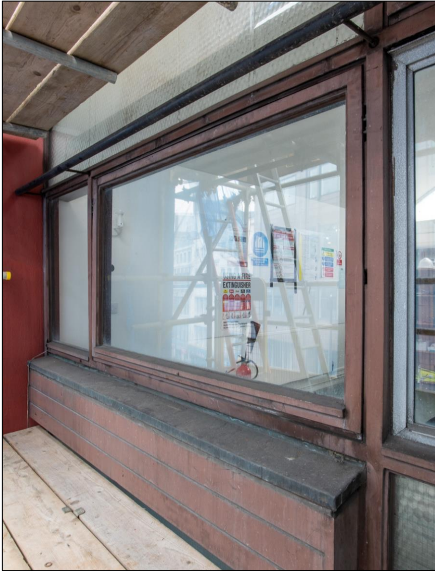
Figure 19. Projecting bookshelf cladded with groove timber boards, looking northeast
