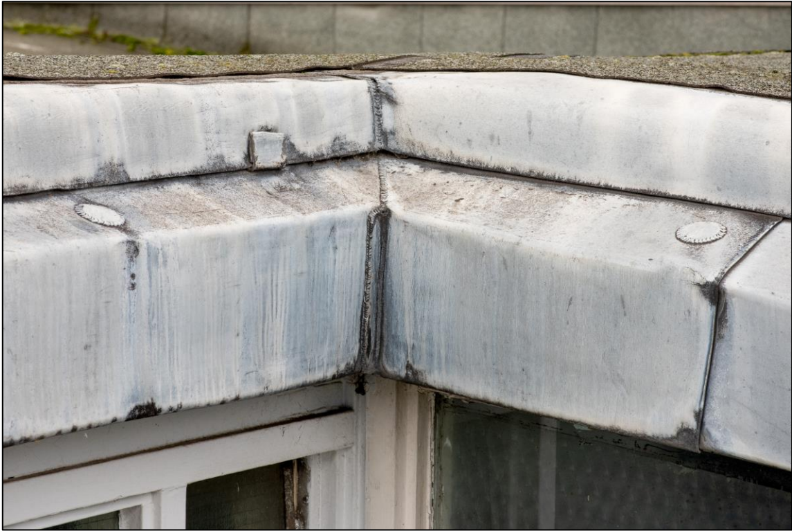
Figure 29. Lead flashing at the edge of building roof above fanlight and bathroom window, looking southwest
