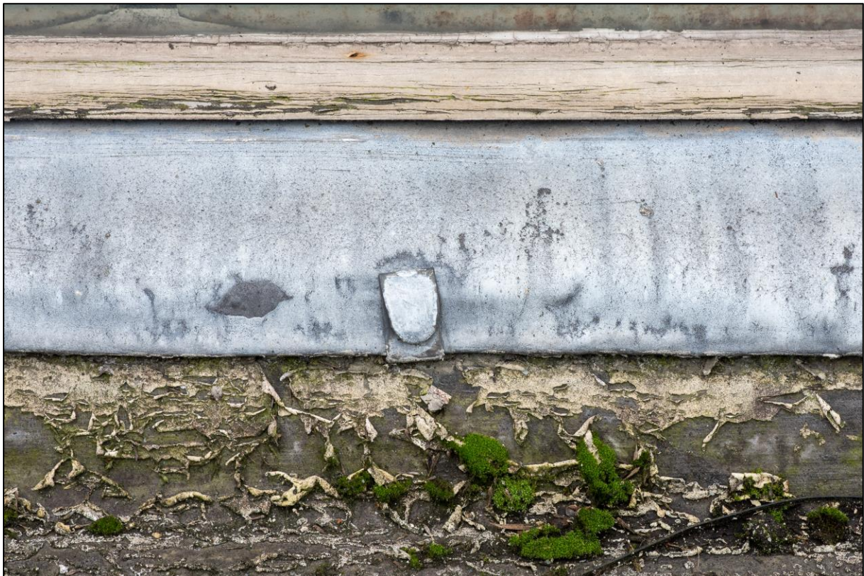
Figure 28. Lead flashing at the bottom part of the fanlight, looking west
