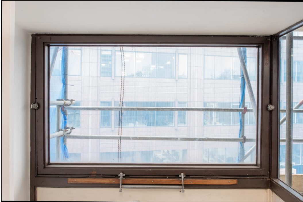
Figure 8. Pivoting window of projecting part, facing Goswell Road, looking west
