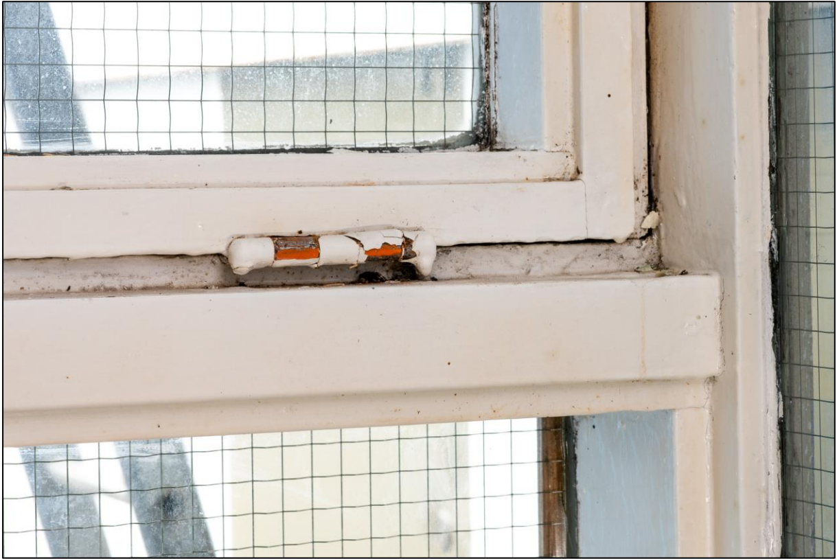
Figure 35. Brass butt hinges of low hang kitchen window facing east
