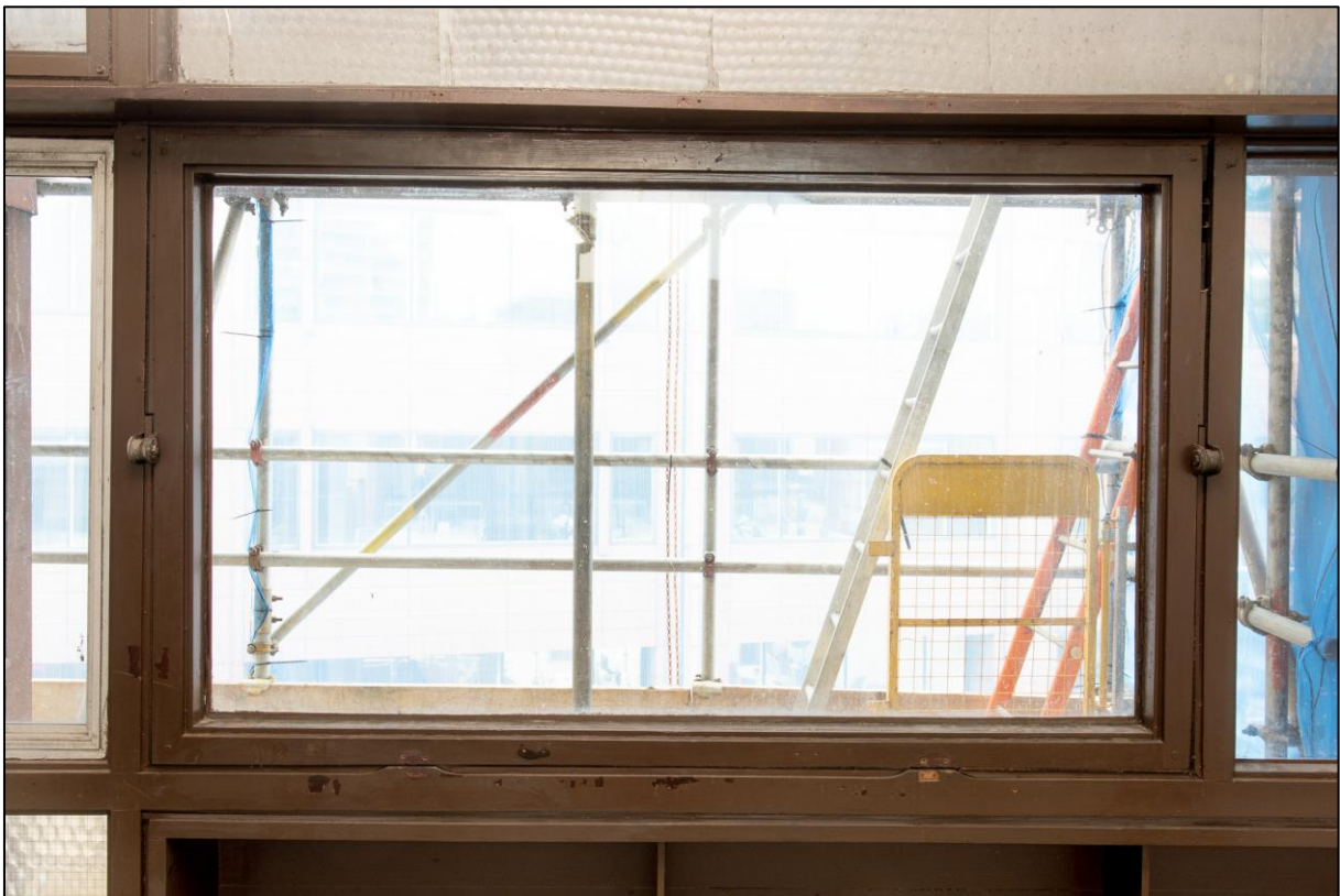
Figure 16. Large central pivoted window, looking west
