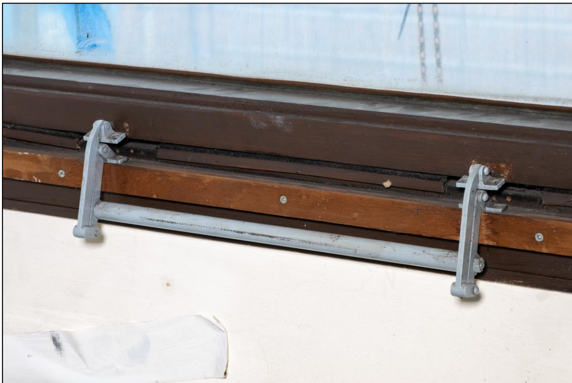
Figure 21. Pivot window handle located on the bottom part of the pivoted window of the projecting south part of the window
