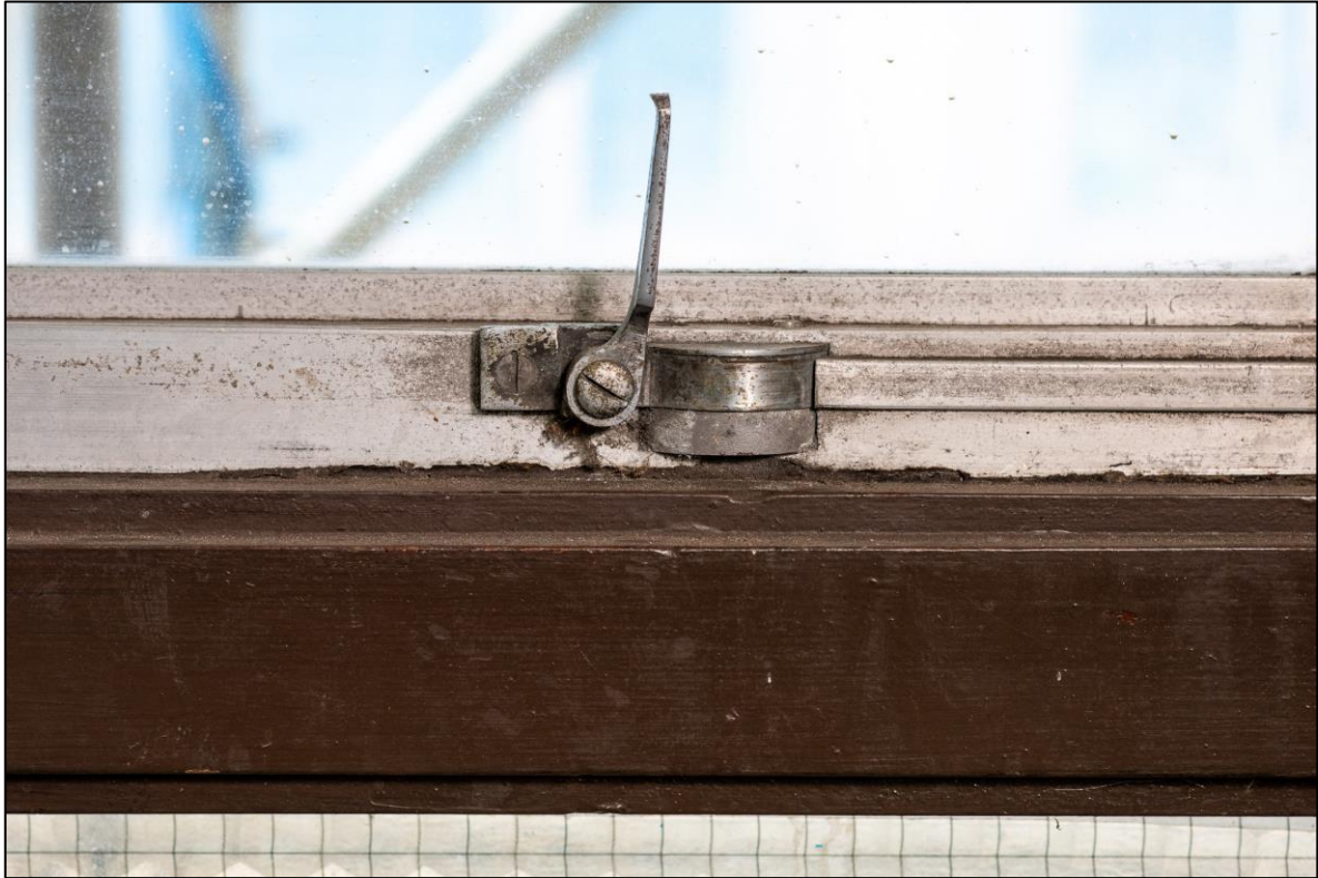
Figure 22. Bottom pivot hinge of aluminium pivoted window
