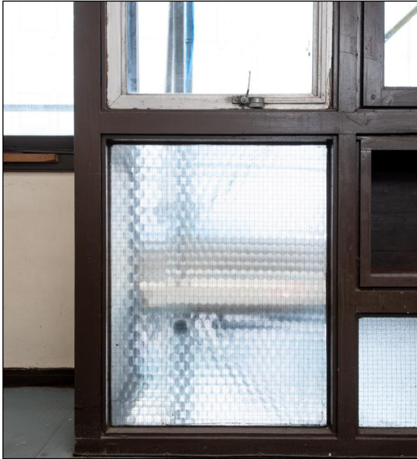
Figure 15. Fixed window with reinforced, translucent glass below the aluminium pivoted window, looking west
